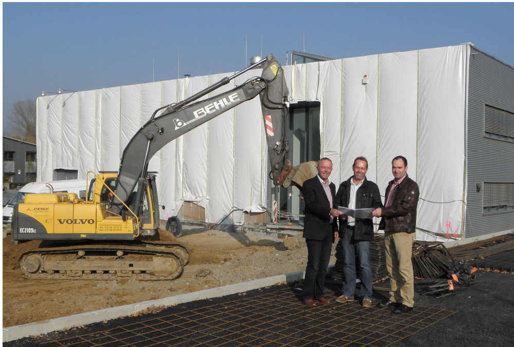
Building contractors and Managing Directors of ENGEL automation and ENGEL in Germany Jörg Fuhrmann (right) and Rolf Sass (left) with the architect Bernd Neuhaus.
