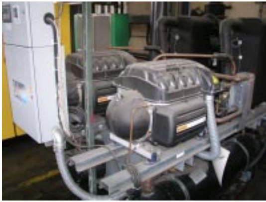
Oil-free compressors from Danfoss Turboacor have only one major moving part - the compressor shaft.
